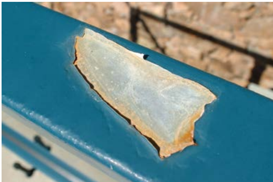
(All images) Delamination coating failure of epoxy/polyurethane duplex coatings on hot dip galvanized surfaces resulting in the accumulation of zinc corrosion products
